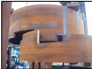
Test Cut - Onshore
