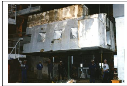
Reinforced Concrete Slab 9.52m x 3.14m x 2.57m 2
