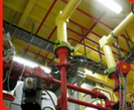
Successfully unblocked cement from 4" 22kpsi cement lines whilst rig was operational
