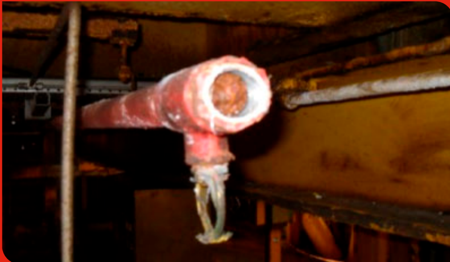
Removal of corrosion and scale deposits from firewater deluge pipework
