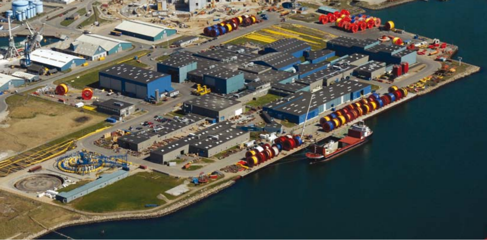
The manufacturing facilities in Kalundborg occupy a total site of 150,000 m 2 , of which 45,000 m 2 is under roof. We have our own quayside with water depths ranging from 7 m to 10 m.
