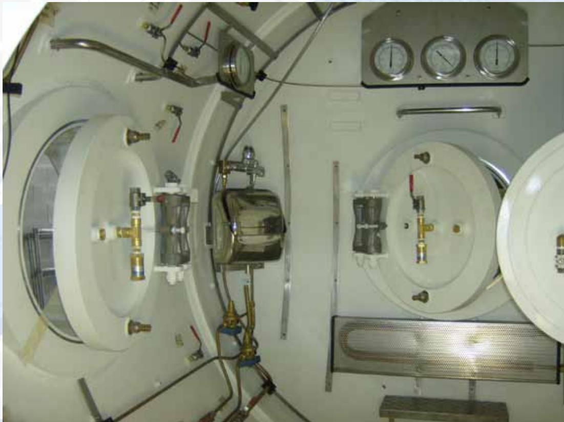
Picture2. 6 - Man Decompression Chamber Internal
