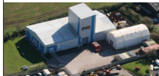
Oil States MCS facility, Barrow-in-Furness
