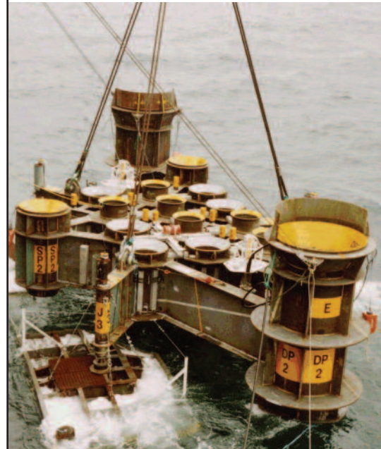
Swaged pile on pre-drilling template
