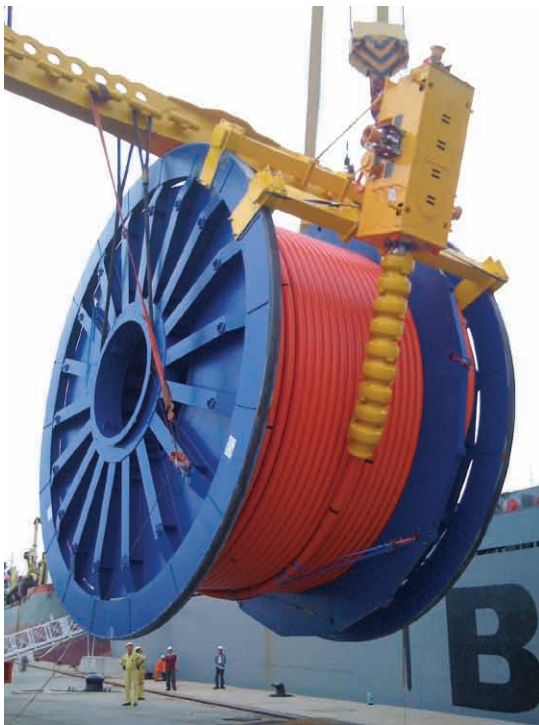
Van Gogh Subsea Umbilical Termination Load Out on 9.2m Reel
